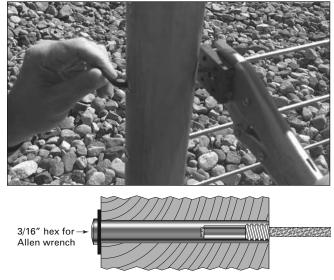
The swaging stud will be pulled into the Receiver by rotating the Receiver clockwise.
