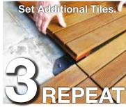
During installation, use the entire connector; use halves or quartered tile connectors on hidden and exposed edges including corners. Use the edge of the spacer to provide a gap between your new tiled deck and any adjacent structure such as a house, fence, or wall.
